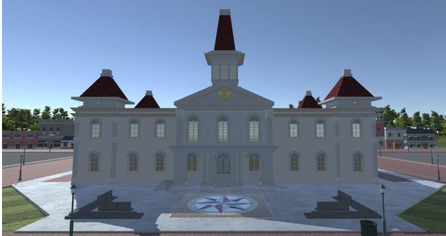
Figure 5 Courthouse – Side C (Unity View)
